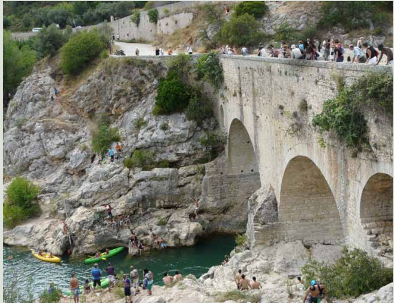
Picture 17. The Diabole de Saint-Jean-de-Fos Bridge is part of an itinerary to discover the A75 motorway.
