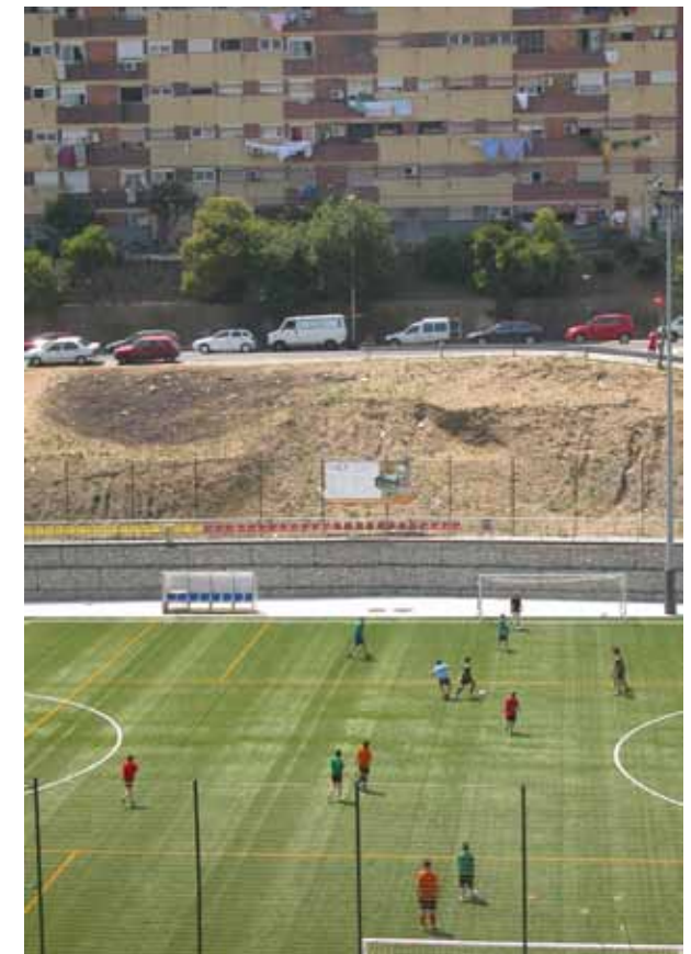
Picture 21. On a local scale, it is easier to find specific solutions to aspects that condition the quality of the landscape, such as making the facilities and infrastructure blend in with certain spaces.
