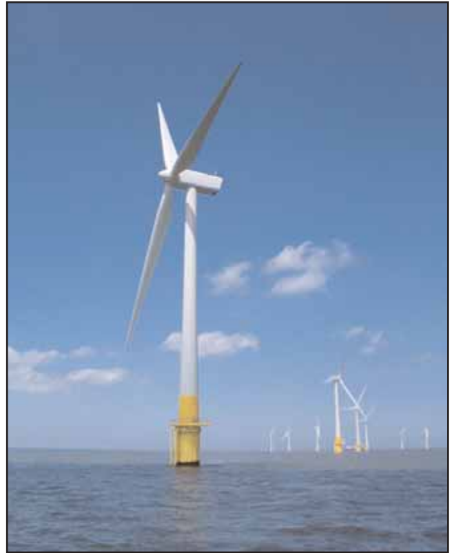
Figure A1: Scroby Sands Offshore Wind Farm
