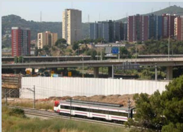
Picture 66. Montcada gorge is one of the main entrances to the city of Barcelona.
