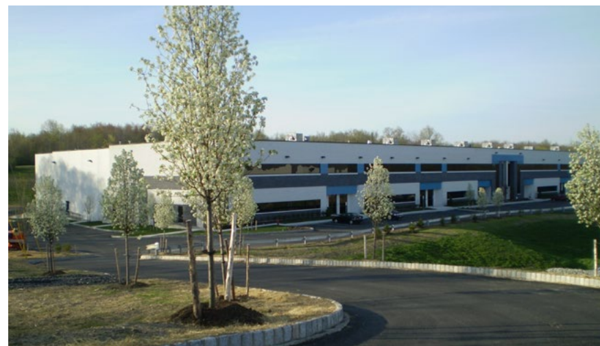
Quickway Industrial Park Site Development (USA). © Tectonic Engineering Consultants, Geologists & Land Surveyors, D.P.C.
