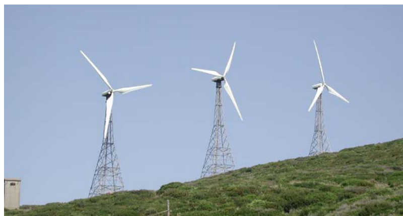
3 bladed turbines on lattice towers
