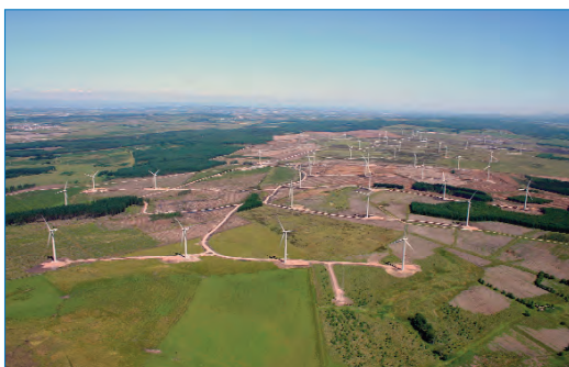
A large windfarm in a large scale, open landscape.
