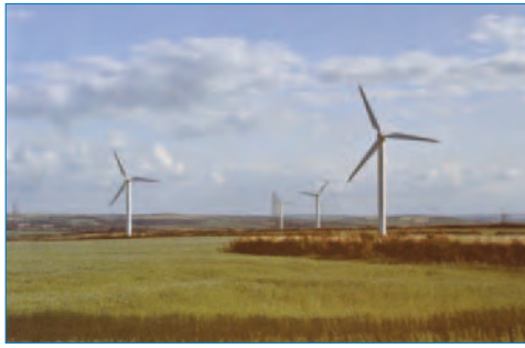
Informal layout. However regular spacing between wind turbines and direct link to landscape pattern gives layout visible rationale and sense of order.
