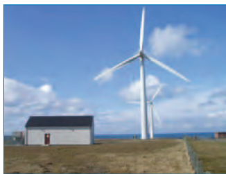
Small windfarm substation
