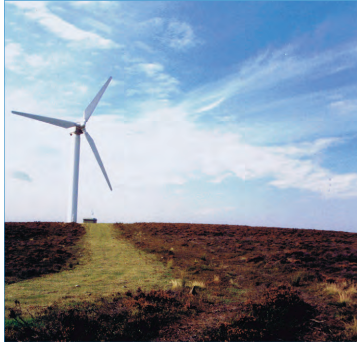
Partial restoration of access tracks to grass
